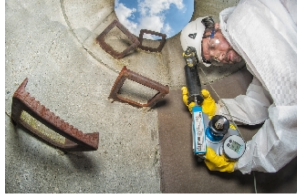
Tensile adhesion test on a coated manhole
