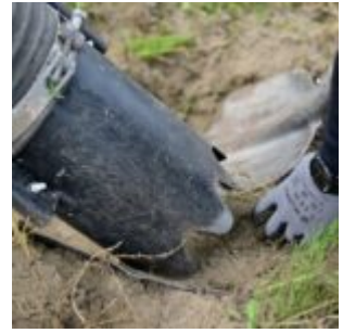
Tree roots are cleared with suction excavators, shovels and by hand.
