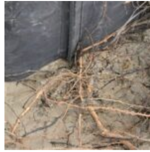
Protective mat to stop roots
