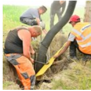
Roots and sewer pipes are excavated with great patience and sensitivity.
