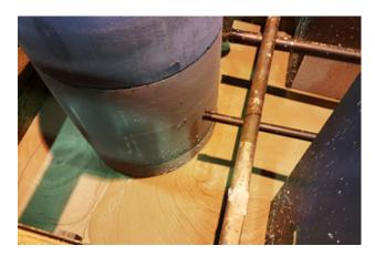
Construction of the 1:1 scale simulated excavations in the test pit: five concrete manhole shafts, five plastic manhole shafts, five sewer pipes, five crossing pipes, ten shoring boxes — and 30 tons of steel to make the trench walls.
