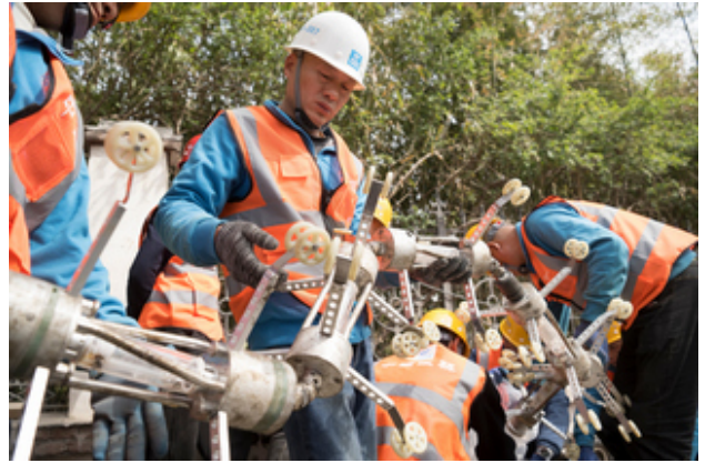
CIPP liner construction site in China
