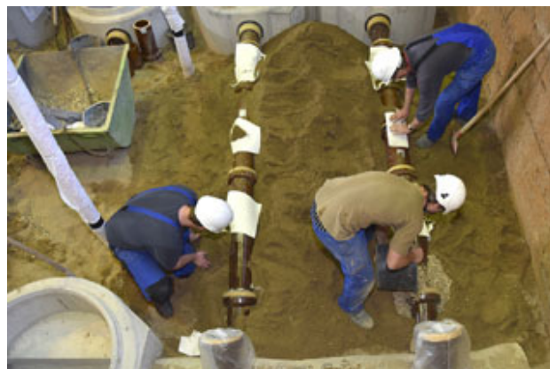
Defined damages: preparing the test rigs
