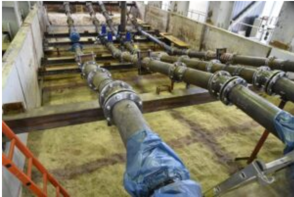
Experimental setup of pressure sewer pipes in the IKT large 1:1 scale test facility
