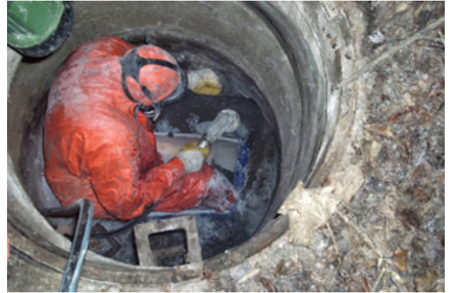
CIPP liner: Taking a sample in a manhole
