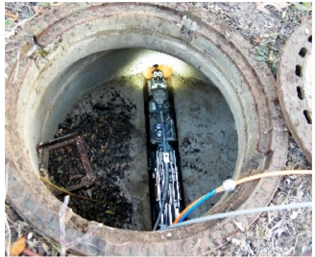
Sewer camera in use
