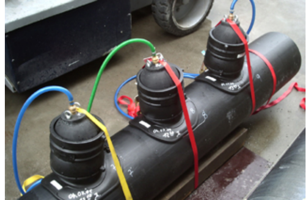
Testing sewer lateral saddles
