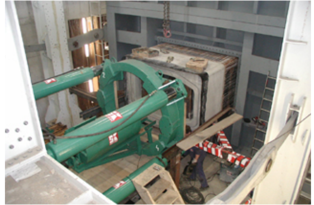
IKT tests jacking pipe with rectangular cross-section in its large-scale test rig
