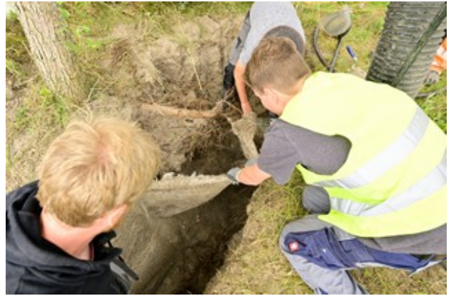
Root protection mat installed in the ground is removed.
